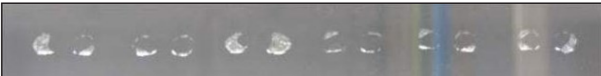
Figure 43 Cracks in glass caused by soldered connectors as visible from the outside face of the product (ACEA et al. 2009)
